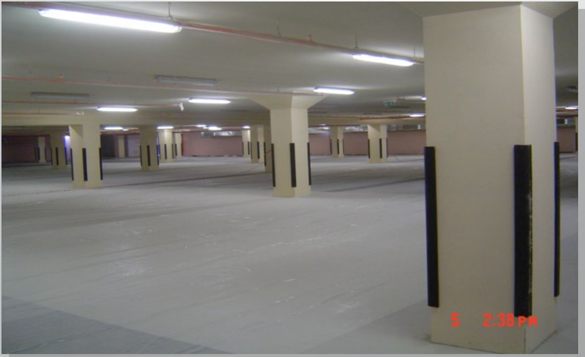
Car Parking Garages @ Jumeriah Lake Towers
